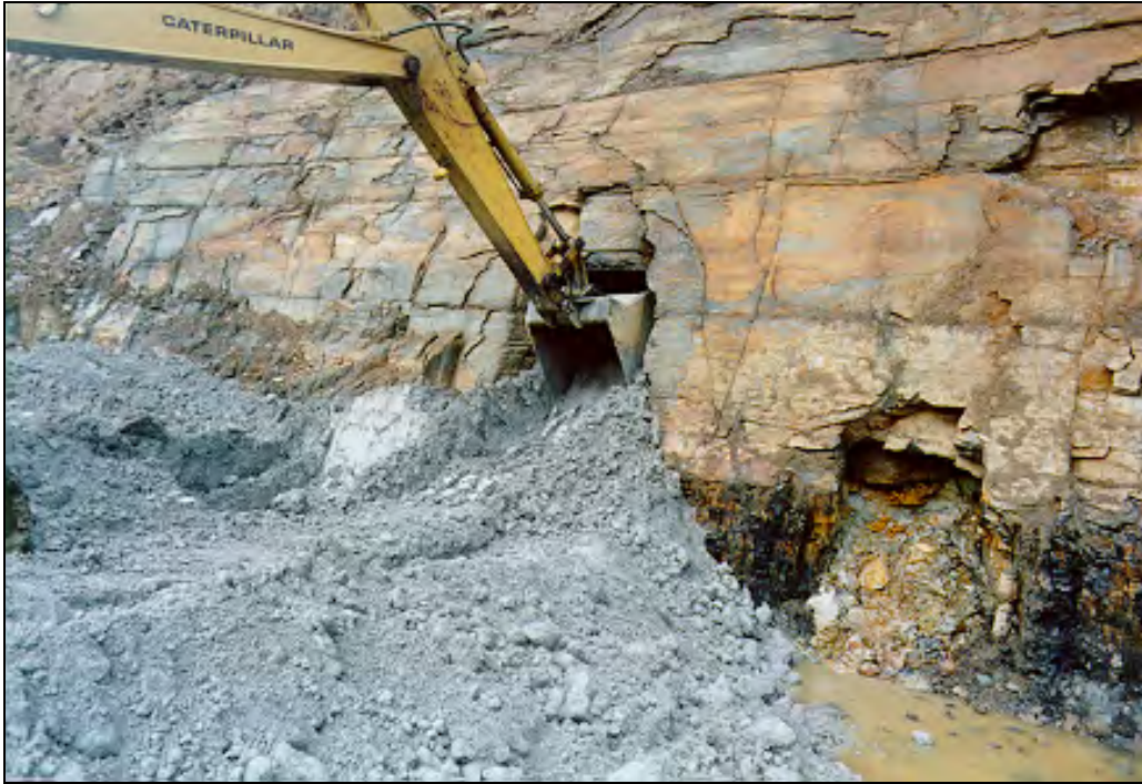
Figure 42 – Broken Aro Project, using a backhoe to fill mine openings.
