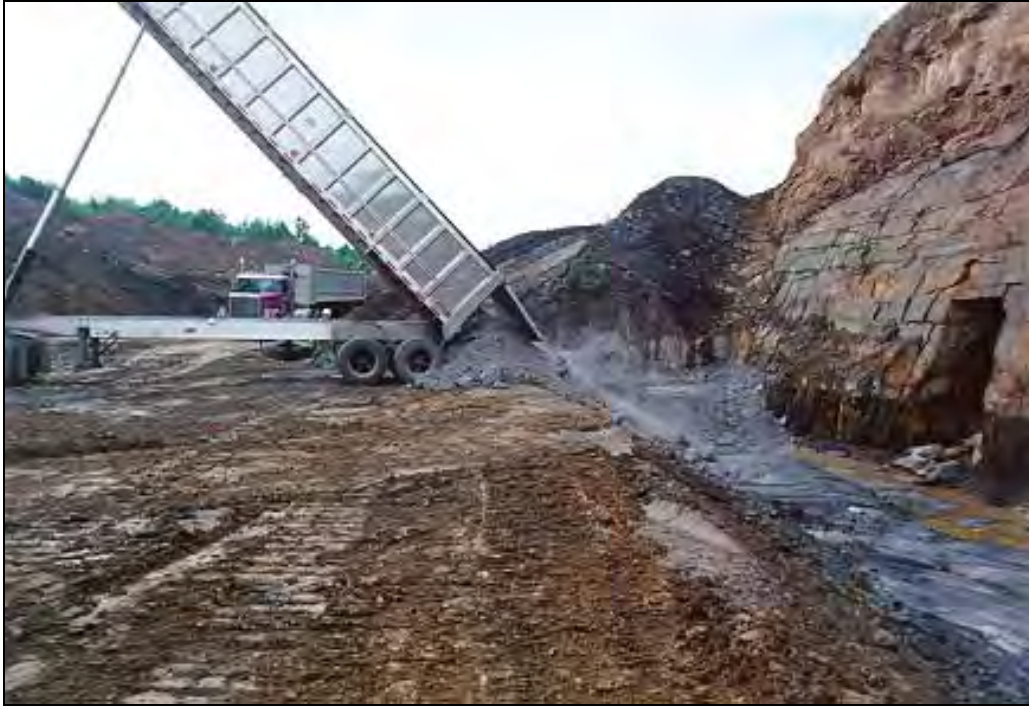
Figure 39 – Broken Aro Project, dumping FGD in trench against highwall.
