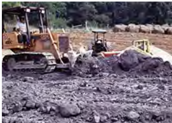
Figure 5. Spreading of FGD
