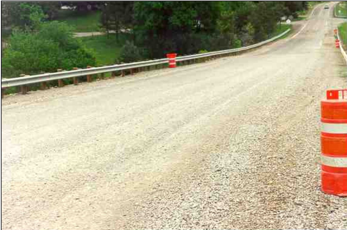
Figure 33 – SR 541 after PFBC placement and before paving.
