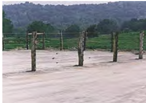
Figure 7. Completed FGD pad
