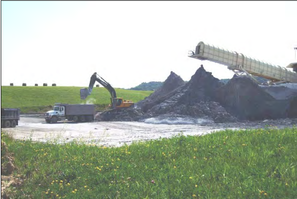
Figure 8 – FGD Storage Pad.
