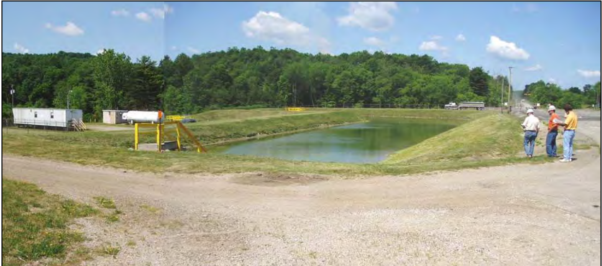
Figure 20 – Treatment ponds and facility, AEP Landfill.
