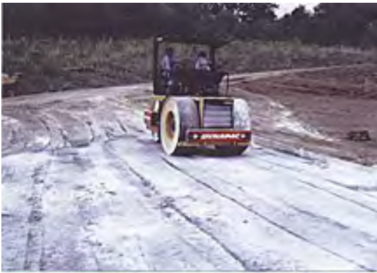
Figure 6. Compaction of FGD
