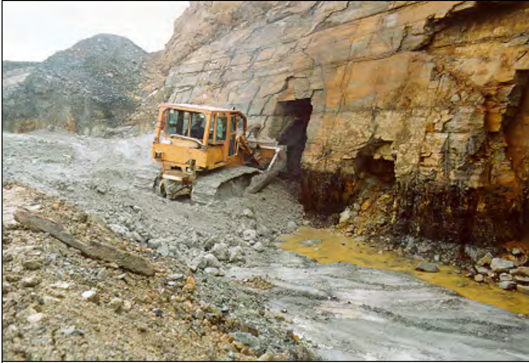
Figure 41 – Broken Aro Project, compacting FGD material with dozer.
