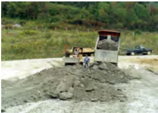
Figure 4. Delivery of FGD
