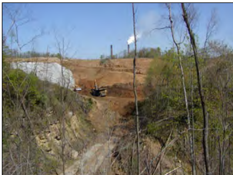
Figure 29 – FGD material being deposited on site.
