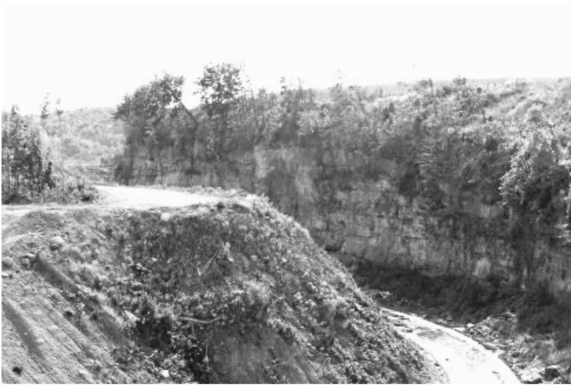
Figure 1. Abandoned mine land with exposed highwall and acidic seepage at base of highwall prior to backfilling and reclamation using FGD residue.
