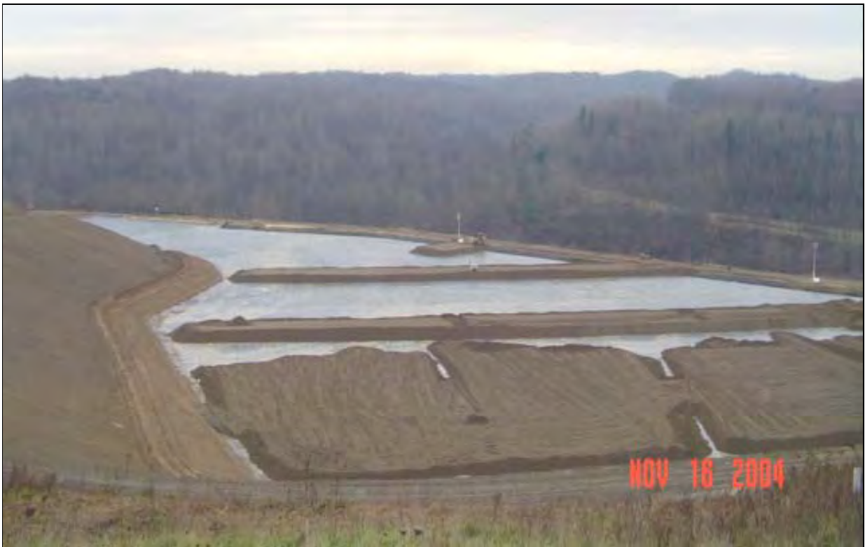
Figure 19 – Leachate Collection System Drainage Layer (Sand), Phase A Area.
