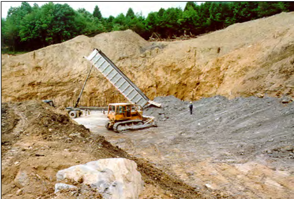
Figure 44 – Broken Aro Project, the final grade is sloped to shed water.
