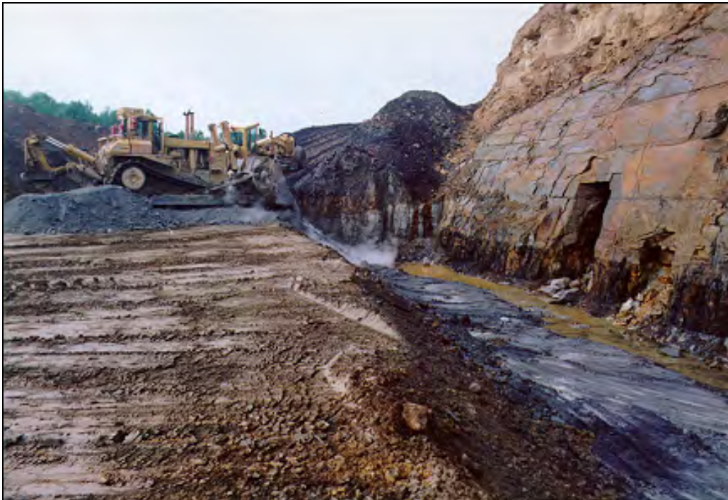
Figure 40 – Broken Aro Project, moving and blending FGD with dozer.
