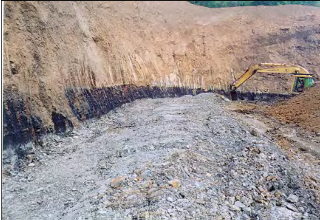
Figure 43 – Broken Aro Project, the first lift is nearly complete.
