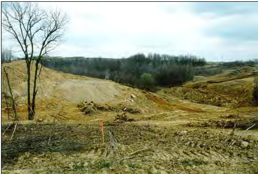
Figure 38 – Broken Aro Project, grubbing and preparation of site.
