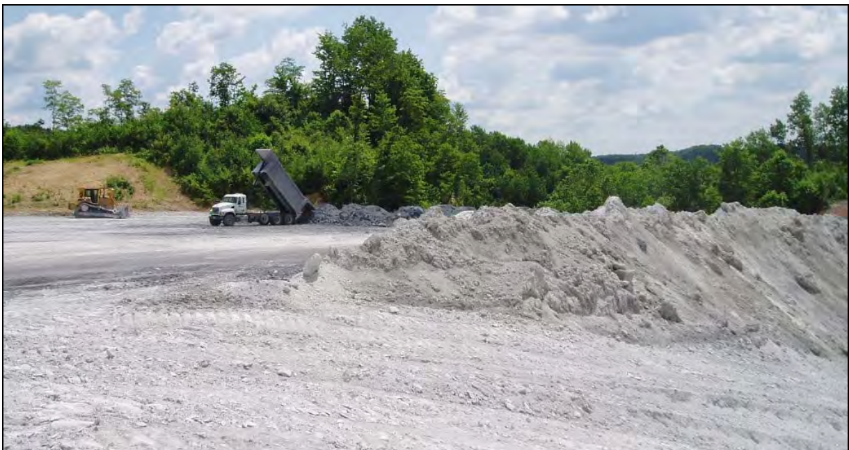
Figure 31 – Unloading FGD material to be spread out.
