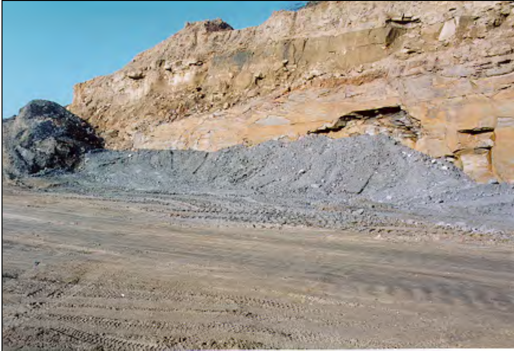
Figure 45 – Broken Aro Project, the FGD ready for backfilling and reclaiming.
