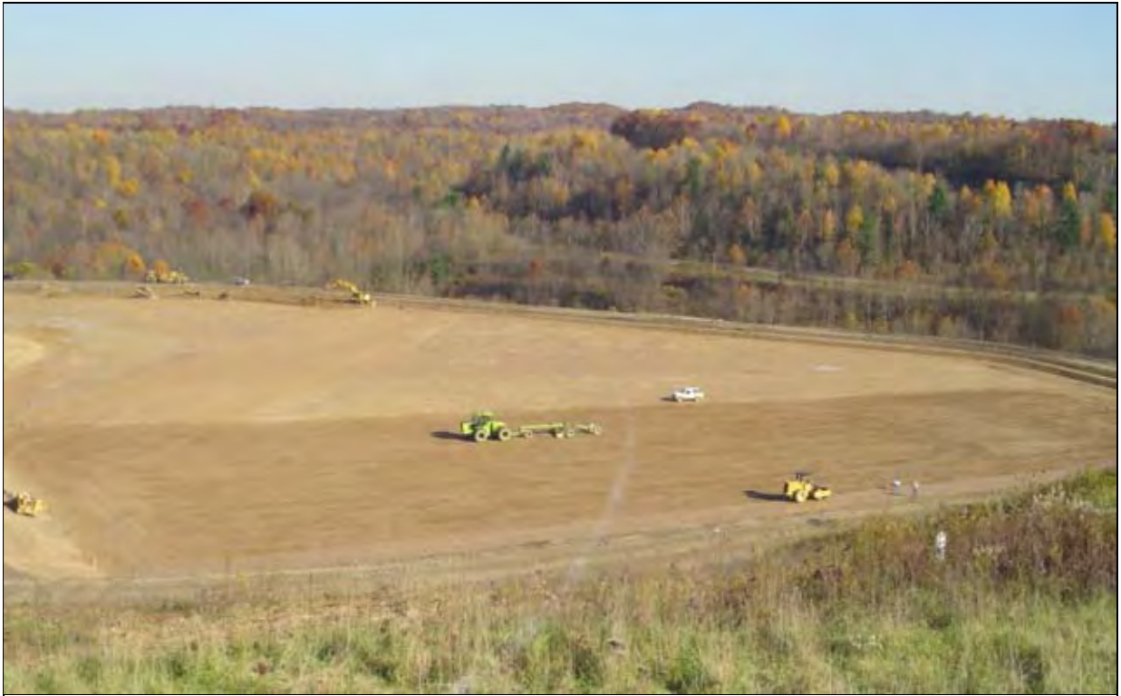
Figure 16 – Recompacted Soil Liner, Phase A Area.
