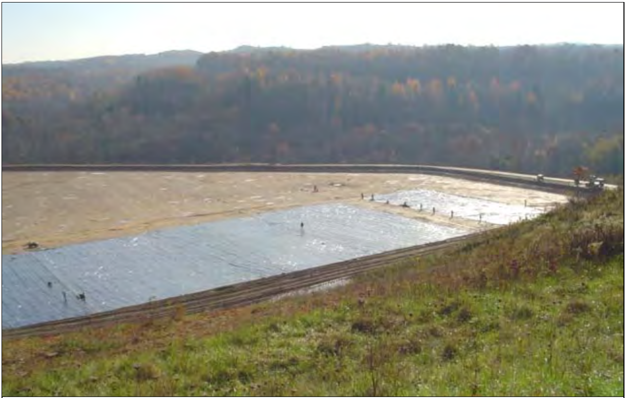
Figure 17 – Geomembrane Liner Installation, Phase A Area.
