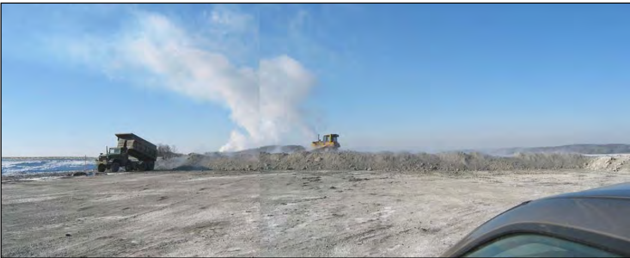
Figure 13 – Placing and spreading FGD ash, AEP Landfill.
