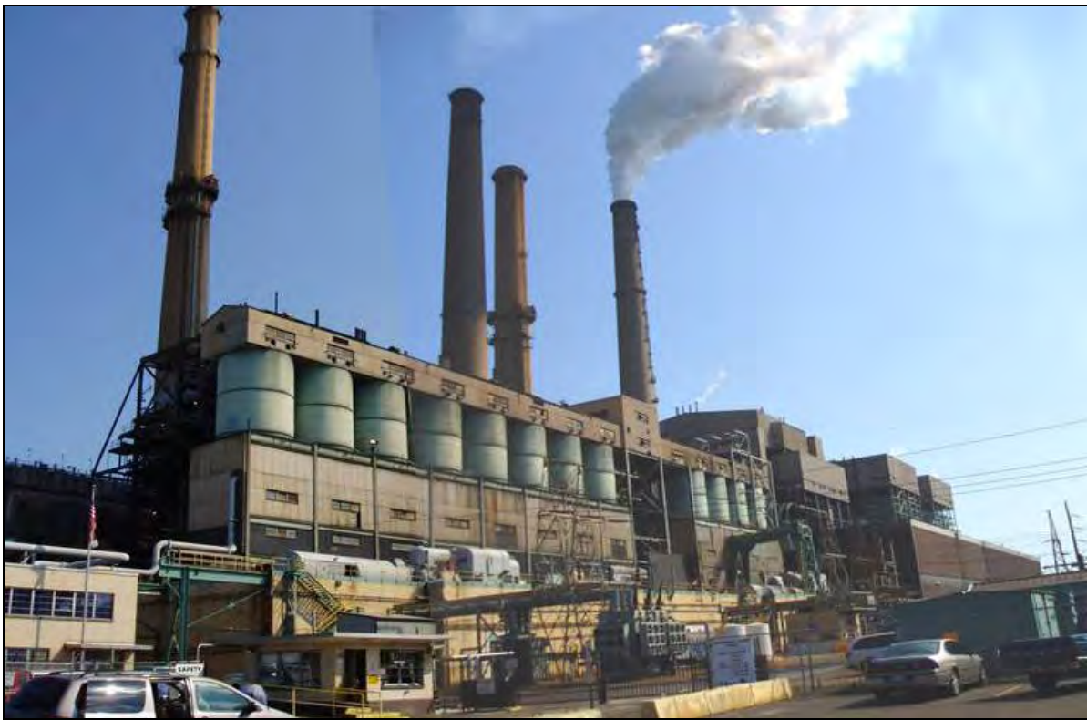
Figure 4 - Closer view of the Conesville Power Plant from the main gate.
